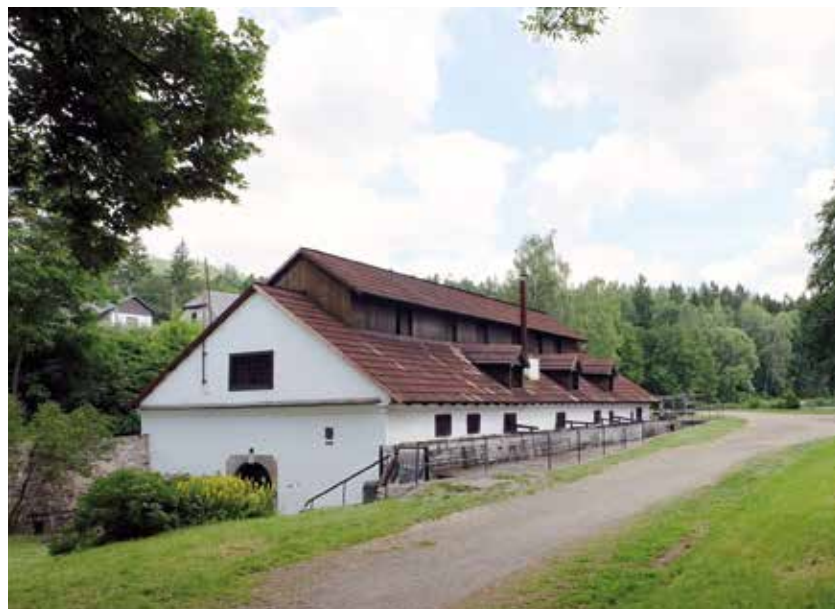
Dobřív, hammer mill, Dr. Bohuslav Horák Museum, a branch of the West Bohemian Museum in Plzeň (Západočeské muzeum v Plzni). The hammer in Dobřív (national cultural monument), featuring complete functioning machinery enabling technologies to be presented to visitors. Photograph Ondřej Merta, 2016.
