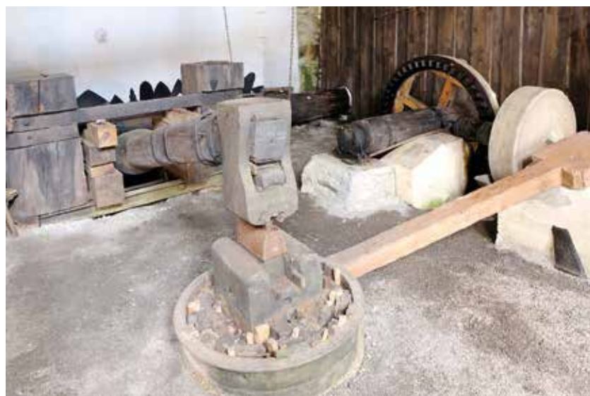
Trhové Sviny, Bušek hammer mill. An authentic installation – a hammer and a grinding machine powered by water wheels. Photograph Ondřej Merta, 2016.
